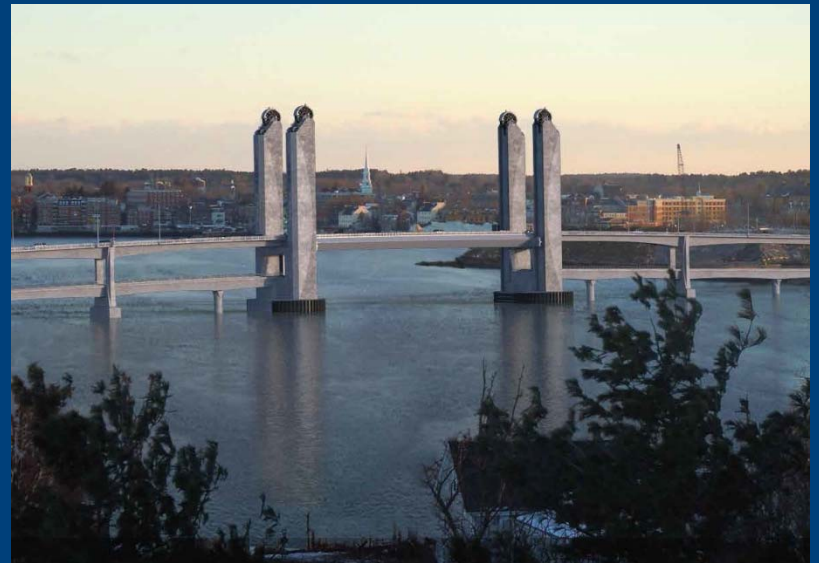
New ME-NH Sarah Long Bridge (opening October 2017)
